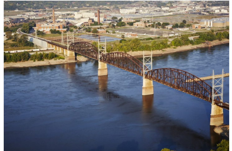
The Merchant's Rail Bridge is a major piece of infrastructure that regional industry leaders prioritized for investment via the St. Louis Regional Freightway. Source: St. Louis Regional Freightway.
